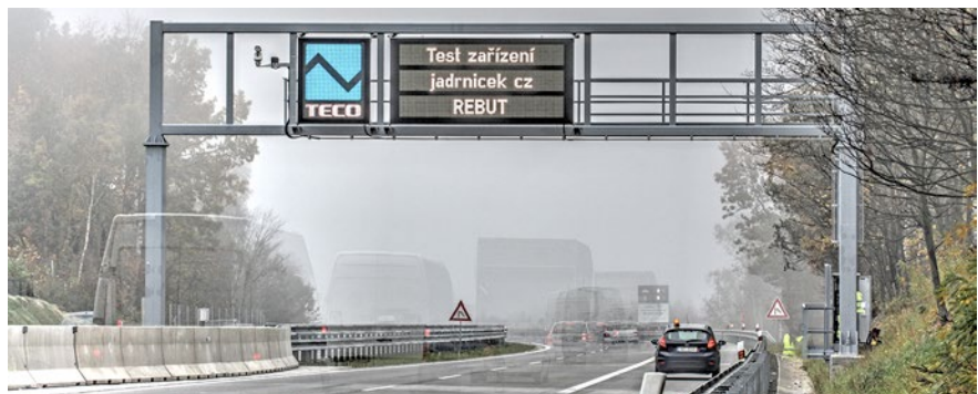
Fig. On three portals/boards namely at the 33.6 km, 54.4 km and 55.2 km of the D1 highway you can see Tecomat Foxtrot systems working above the heads of passing drivers. These are used as communication units processing commands from the National Information Center. Photo by: Vit Jadrnicek
