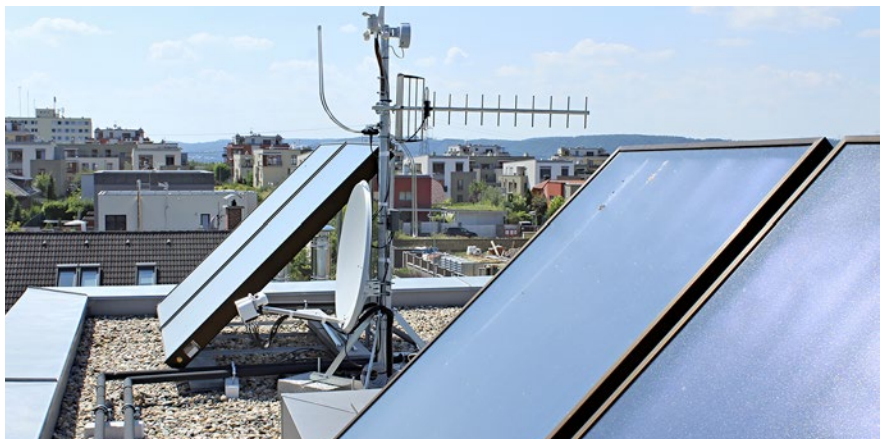
Fig. The roof of the house is an inseparable part of the building control technologies. It actually represents an engineering "room or space" which carries the installed thermal solar panels including weather station and communication antennae which talk with the world.
