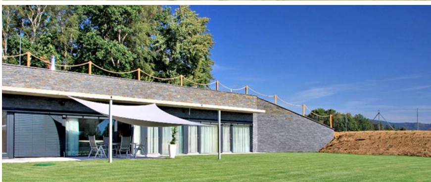
Fig. Houses built by KONHEFR use Tecomat Foxtrot to automatically control their infrastructure
