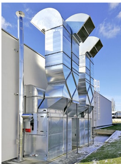
Fig. Argus heaters and air-conditioning system from CIC Hrebec controlled by Foxtrot are other technologies which affect the inner climate of the building.
