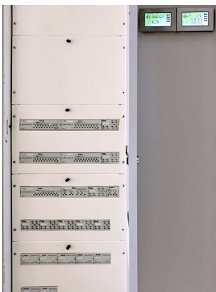
Fig. Electrical cabinet with peripherals is connected to the center with double-wire CIB® bus. High capacity modules offering 6 to 32 inputs/outputs are used here. The modules are placed elegantly and covered in regular power cabinets on the DIN rail, in a similar way as circuit breakers for example. When in manual mode, each circuit may be controlled from the front panels independently. This is a handy feature used when the system is being put into operation, during service checks or in an emergency situation. There are also two displays fixed on the wall offering comfortable control features and which are also displayed on a remote tablet, smartphone or PC.
