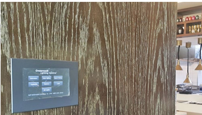
Fig. Built-in design of the ID-32 panel which is the central location used to control the lighting system and to configure the desired scenes.
