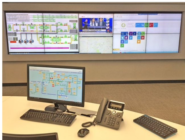
Pic 4: Reliance SCADA, AVE and MARUSHKA GIS are displayed on the big LED wall in Baskentgaz
