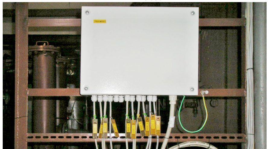
Fig. This picture shows the data collection system. Data are received from the modernized oil management system overseen by Tecomat TC 700.
