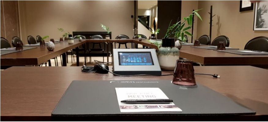
Fig. the control panel in each hall is connected to Foxtrot system which allows the operator to access all functions and set parameters in the hall.
