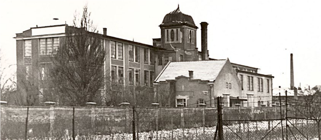
Fig. After 1945 the company was nationalized and until 1993 the company was known as Tesla Kolin. The original building No. 260 was newly marked as M1 and underwent several reconstructions.
