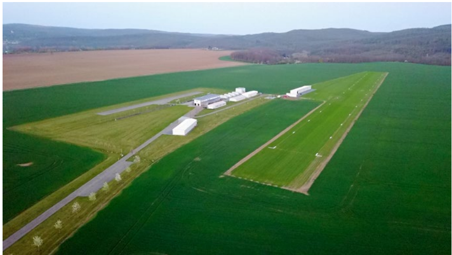
Fig. A complete view of the airport before sunset as seen from a drone sent to take the pictures for this article. In the background you see a small concrete runway for model airplanes and at the front to the right there is a large grass-covered runway for sport and acrobatic airplanes.
