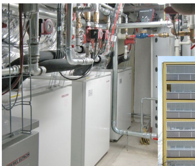
Fig. An apartment building in Francouzská street in Koprivnice uses a cascade of four heat pumps Stiebel Eltron "air-water", type WPL 23E. This system has demonstrated over the past 7 years that savings of 50% are possible when compared with regular central heating system
