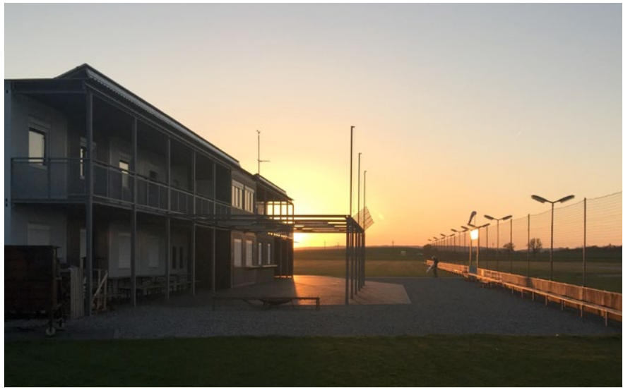
Fig. Night covering the central area with a tribune and commercial building, which also includes a small dormitory – also controlled by Tecomat Foxtrot.
