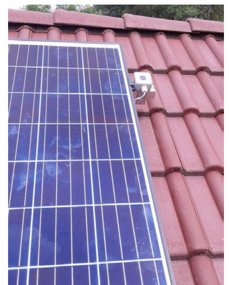
Fig. Foxtrot integrated in the Airsun system monitors the level of solar radiation using special sensor on CIB bus.
