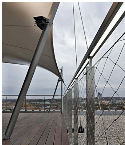
Fig. 6 the terrace is protected with a tensioned canvas roofing. the indirect illumination of the roofing and the built-in LED stripes in the lower section of the handrail area create interesting light effects and scenes, particularly at night.
