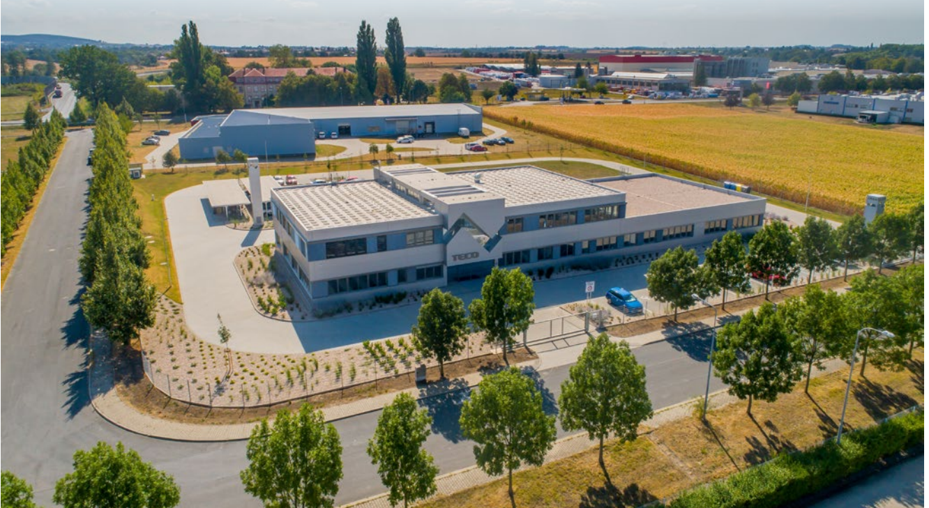
Fig. the new building of Teco a.s. is approximately 1.4 km from the old one towards the east in the industrial zone called Štáralka. the drone view shows that this factory was literally built on a green field and it took only 8 months. Even though the building looks like a silver technical piece, the building is actually green. This is because the building covers 50% of its energy needs for heating and cooling from renewable resources. There are twelve deep drilled wells on the land. Even the rain water collected by the building roof goes to reservoirs below and it is used to water greenery or to flush toilets. the building became fully operational at the end of November 2017, three weeks after the staff moved in.
