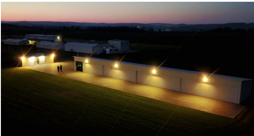
Fig. You may use your mobile phone to remotely control the outdoor or interior lights in the new hangar.
