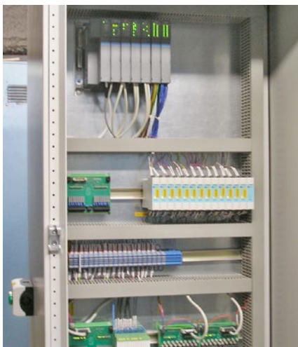
Fig. This picture shows the data collection system. Data are received from the modernized oil management system overseen by Tecomat TC 700.
