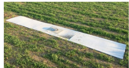
Fig. A detail of the landing runway light installed in the center of a white rectangular with highly reflective surface.
