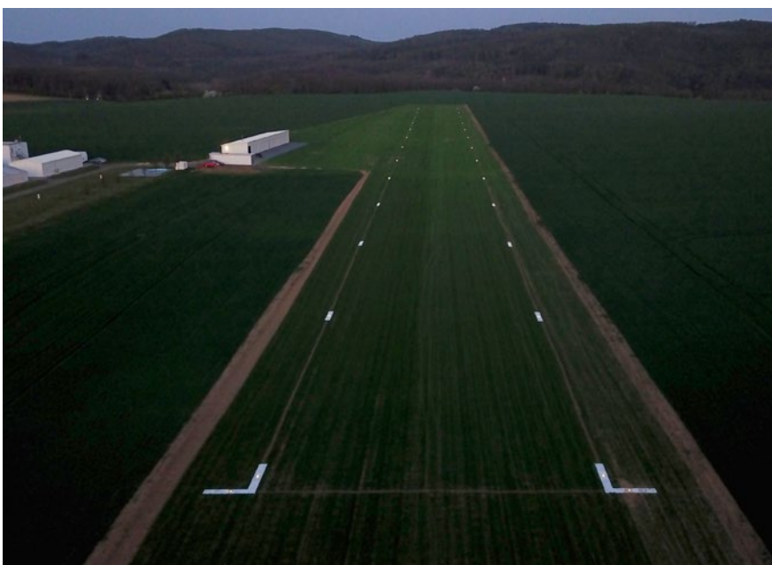
Fig. Runway lights for acrobatic planes may be turned on by the pilot remotely using his own mobile phone and based on his own needs. the signal is received by Foxtrot unit installed in the new hangar.
